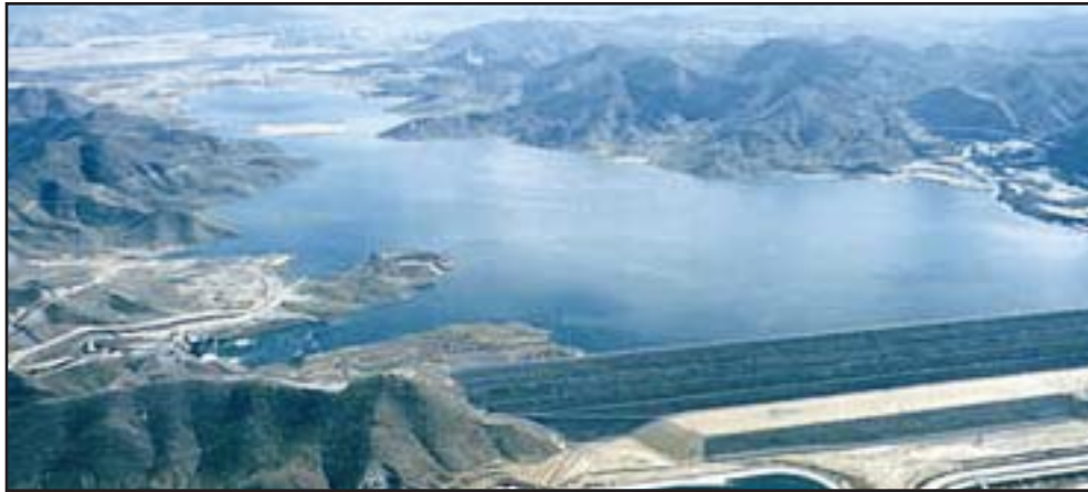
MWD's Diamond Valley Reservoir
